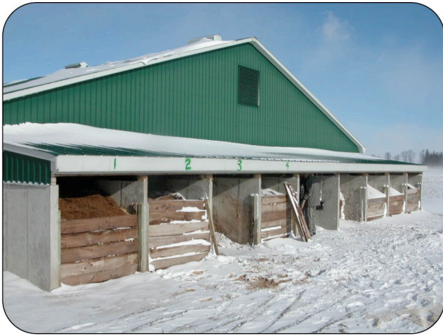
Figure 2. Actual bin system showing two primary and secondary bins, plus bins for finished compost and storage of substrate.
