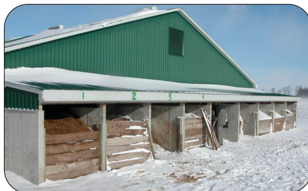
Figure 1. This well-designed bin composter on a swine farm was working well the January day of this photo when the air temperature was -15^{\circ}\text{C} .
