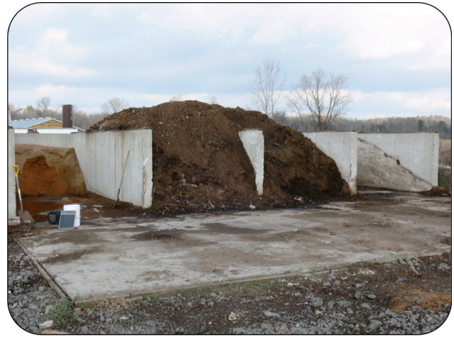
Figure 3. This bin compost system (for swine) has four bins; filling, primary heating, secondary heating and substrate storage. Bins are not normally filled to overflowing. The apron floor area out front encourages clean-up and is sloped away from the bins in all directions. Bin floors are sloped slightly to the back. The operator said he would make the apron area bigger if doing it again.
