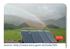
thermal hot water systems in the region. While warmer climates are able to pass water directly through the panel array, Maritime farms are required to use food grade glycol solution to transfer thermal energy from the panel array to a heat exchanger where energy is extracted and stored in a traditional hot water tank until it is required for use.
