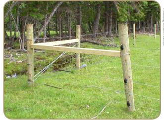
Fig. 1 The "H" brace with tension wire and tension device.
