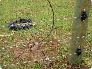
Fig. 4 This figure shows a ground return system with live and ground wires attached to the post. Note the additional ground rod to ensure good grounding.
