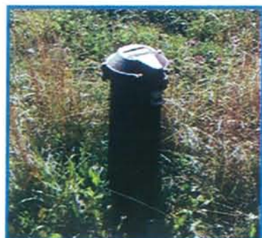
A Drilled Well With an Approved Vermin-proof Vented Pitless Well Cap and At Least 6 inches of Casing Above the Land Surface
