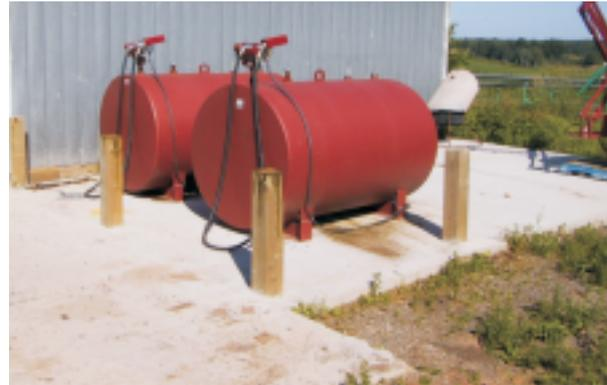
*Fig.1. Fuel tanks on a concrete pad with protective posts.*
